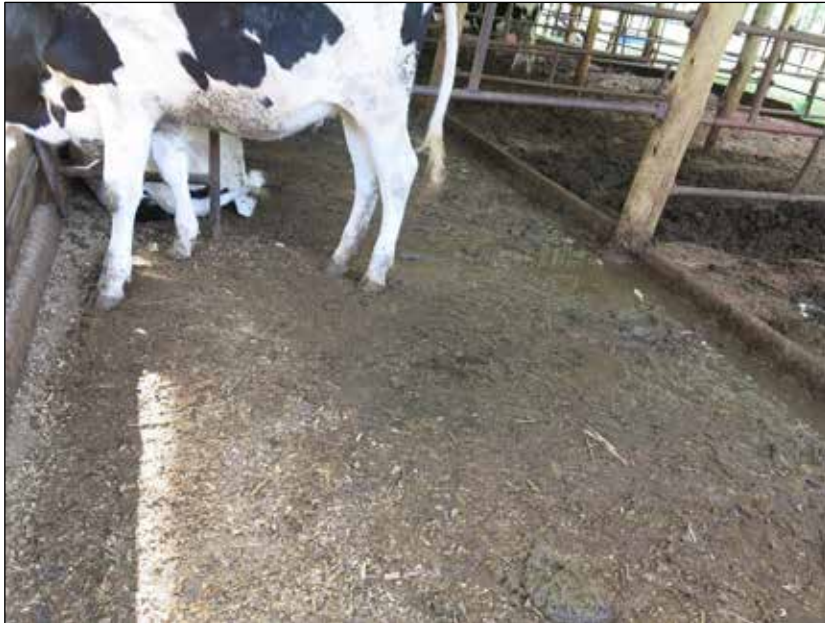
Figure 6. Wet concrete floors Wet concrete floors easily get slippery preventing cows to walk safely and comfortably.
