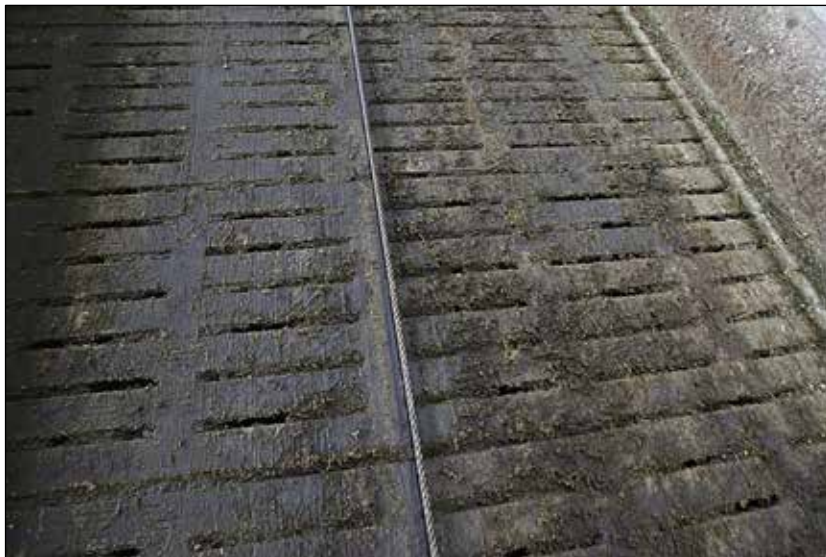
Figure 9. Dry concrete floors
