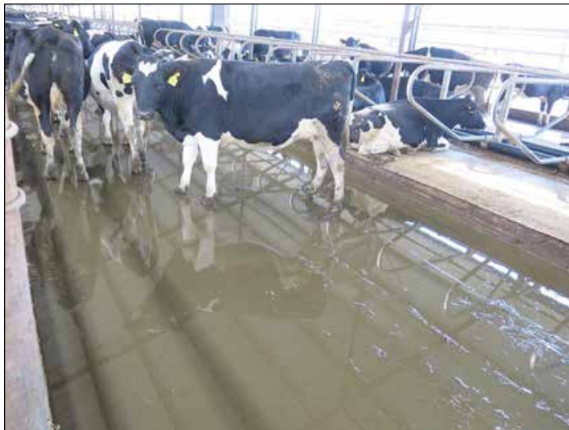
Figure 7. Flat concrete floors Bad Practice: Flat concrete floors (not sloped) remain wet, as urine and other fluids do not run off.
