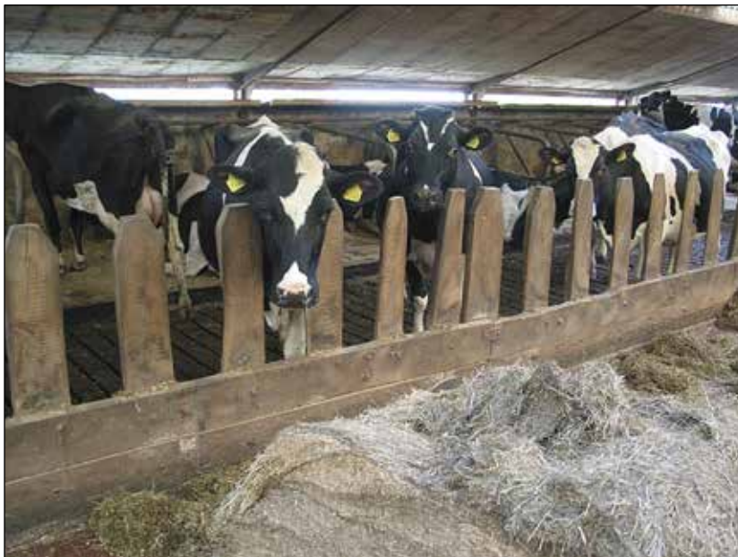
Figure 20. Swedish feed fence from wood The Vetoice/The Friesian Modular Dairy Barn recommends a Swedish feed fence for young stock. Here this feed fence is made of solid wood. Neck opening for young stock: 20 cm.
