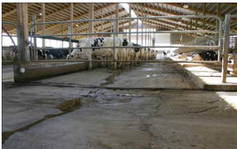
Figure 8. Sloped floors Good Practice: Example of a floor that slopes over lengths and towards its centre. The lowest point should have been further away from the feed fence, so that the eating cows stand as little as possible with their hind feet in manure and urine.
