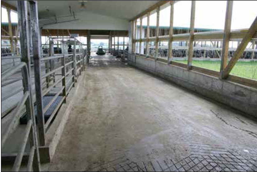
Figure 15. Floors and support posts (2)
