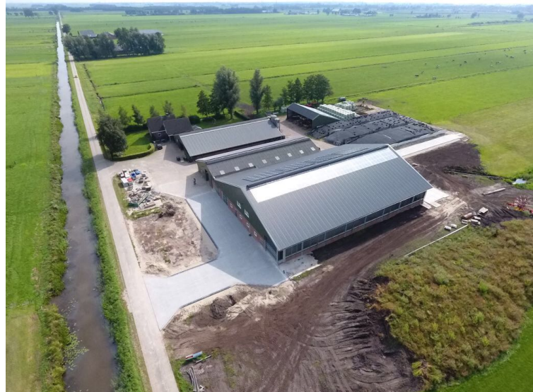
Pic 13: Aerial view of the Bles Dairies farm, Broek
