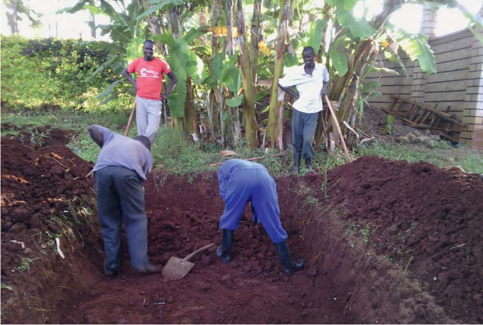
A pit is dug for the silage.
