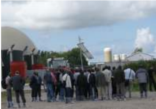
Figure 3: Participants view a huge manure processing and biogas plant at the Dairy
